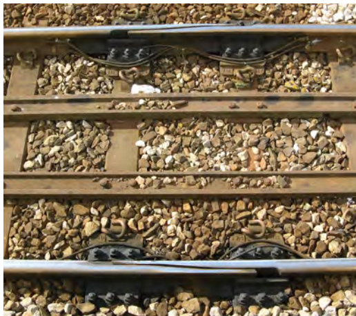
Figure 12.5: This expansion joint allows the length of the rails on either side to expand or contract by several centimeters without losing alignment with each other.[78]
